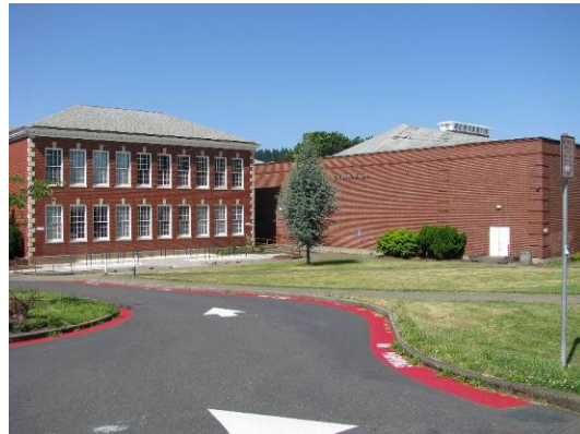
Main building (215A) and new gymnasium addition (215E), looking northeast.
