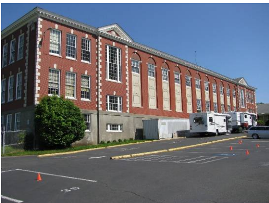
West elevation of former gymnasium (215B).
