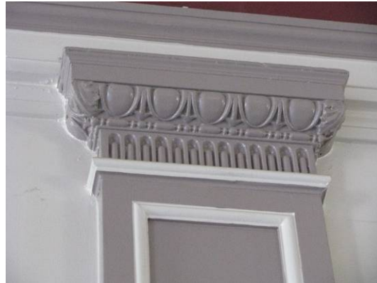
Detail of engaged column capital (215A).
