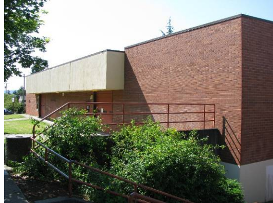
Wood and metal shop building (215F), looking west.
