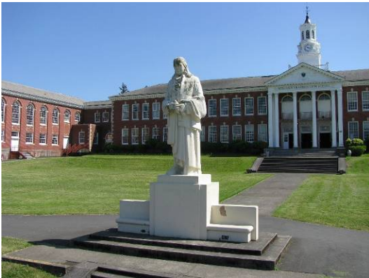
View of Benjamin Franklin statue and main building entrance on north elevation. (215A).
