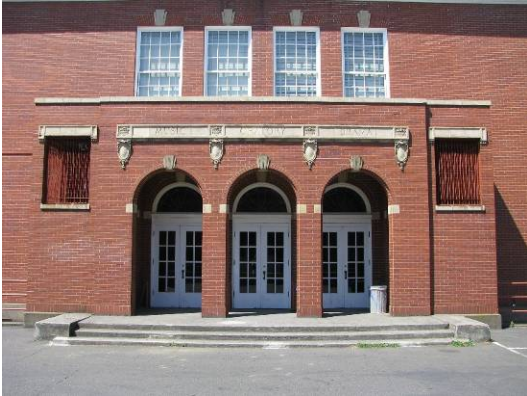
South elevation (main entrance) for auditorium (215C).
